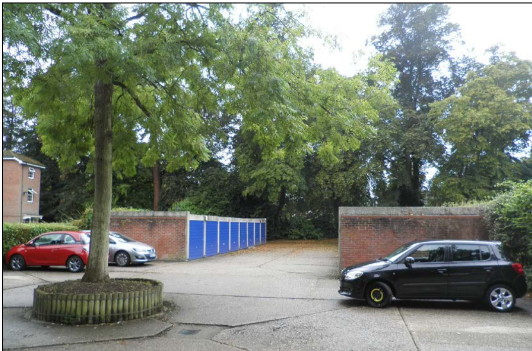
Garage Court/Car Park
